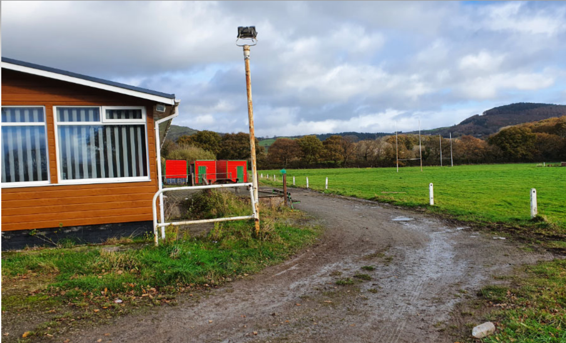
View of existing site
