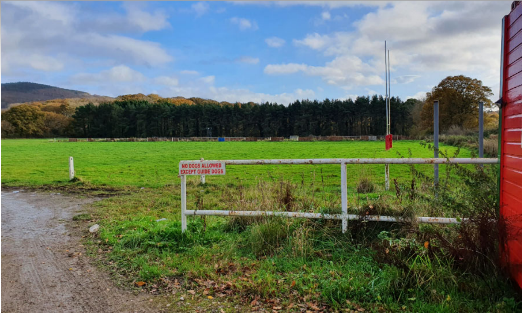
View of existing site
