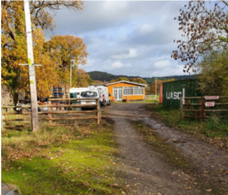
Existing building and approach to playing fields:
